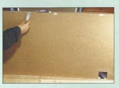
A sheet of fiberboard serves as foundation for the backdrop. Don't forget to cut out the openings for the track with a sharp knife before the backdrop is glued and nailed. The nail holes can be filled (eg, with Revell Plasto) and sanded. The final stage is a thin coat of white glue.
